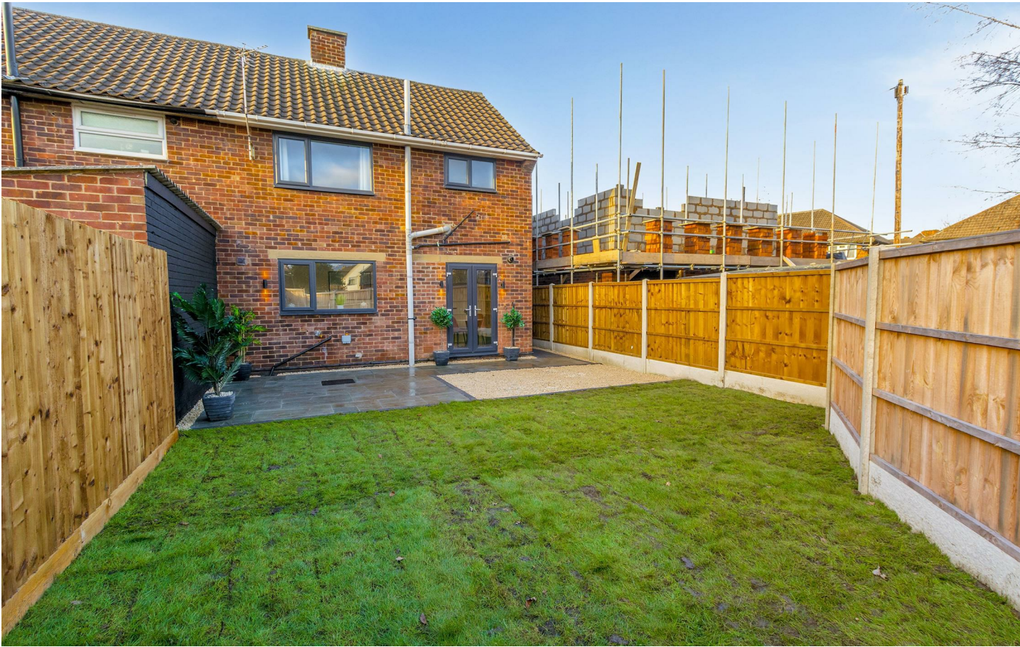
A THREE BEDROOM SEMI DETACHED HOUSE WHICH HAS BEEN REFURBISHED THROUGHOUT.
